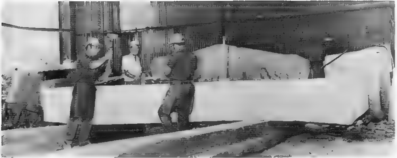
A special crew of Horace and Frankie Bradford, master stone craftsmen, under the direction of Joe B. Davis, background, a retired plant superintendent was hired to cut and polish the granite slabs to the exact dimensions provided by 'Mr. R.C. Christian. Special crews were hired because the project was so demanding that it would disrupt the regular Elberton Granite Finishing Company's production schedule.
